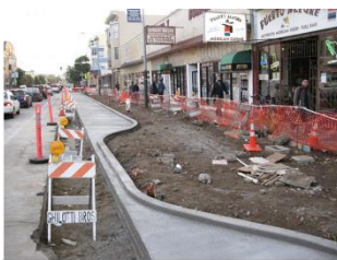
Pedestrian/sidewalk effects typical of side bus lane construction
