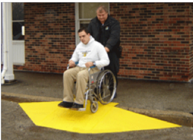
FIGURE 2-25. TEMPORARY CURB RAMP
