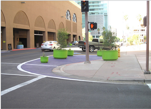
FIGURE 2-4. NON-INFRASTRUCTURE BULB OUTS IN DOWNTOWN PHOENIX
