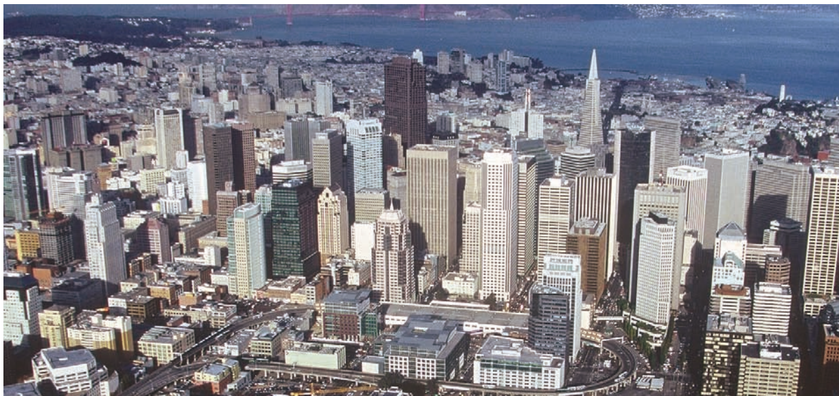
Downtown San Francisco, with the existing Transbay Terminal in the foreground (Source: Transbay Redevelopment Project Area Design for Development )
