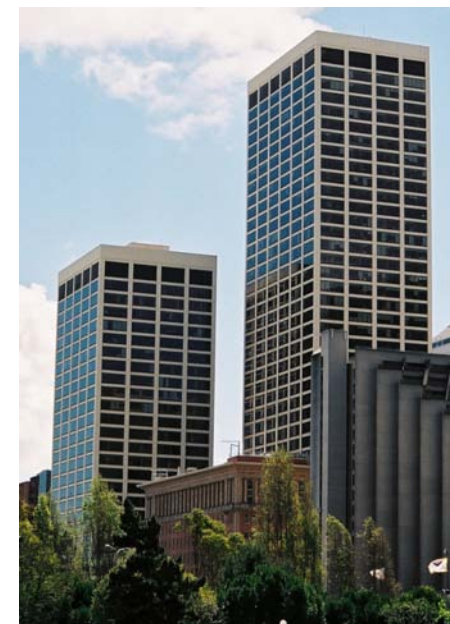
One Market Plaza has a 1.5 MW CHP system
