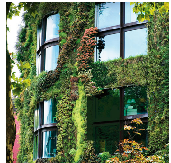
Living walls offer an opportunity to reduce solar gain while adding landscaping to urban areas. Patrick Blanc's innovative vertical gardens, Athenaeum hotel, London (top) and Musée du quai Branly, Paris (bottom).
