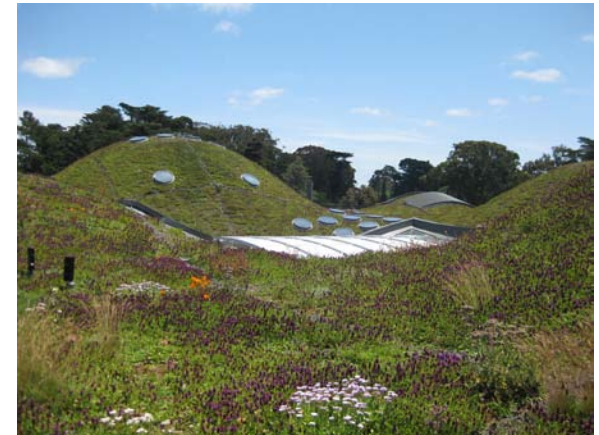
The California Academy of Sciences, a LEED Platinum certified building, incorporates building integrated photovoltaics, natural ventilation, a 2.5 acre green roof and water efficient technologies.
