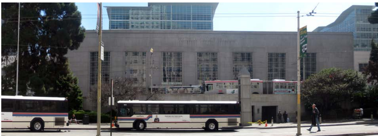
The existing Transbay Terminal is outdated and has a poor relationship to the street.
