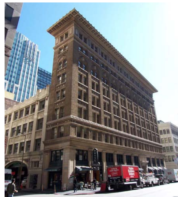
Sharon building (1912), New Montgomery Street (Source: KVP Consulting)
