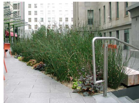
Bioretention planter at Mint Plaza, an example of a water sensitive urban design technique that reduces stormwater runoff, provides habitat, and improves the public realm.
