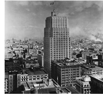
Pacific Telephone and Telegraph Building, 1925 (Source: KVP Consulting)
