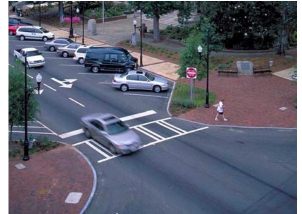
On streets where sidewalks cannot be widened, corner bulbouts can significantly reduce crossing distances.
