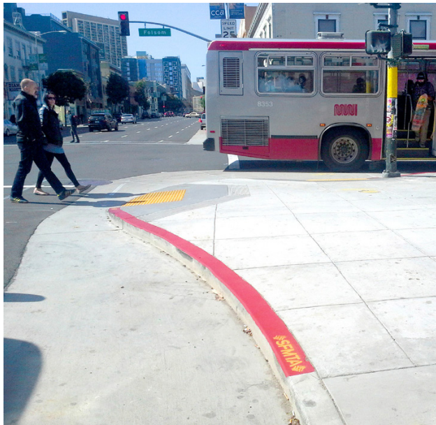
FIGURE 1: EXAMPLE OF A CURB BULB-OUT
