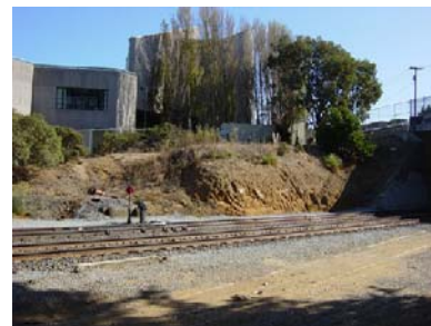
Embankment north of Oakdale Avenue, looking east toward Southeast Community Facility.
