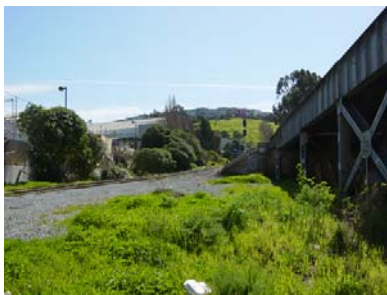
East of Quint Street bridge, looking south toward Oakdale Ave.
