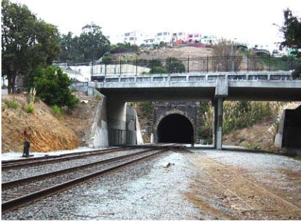
Oakdale Avenue overhead, looking south toward Tunnel 3.
