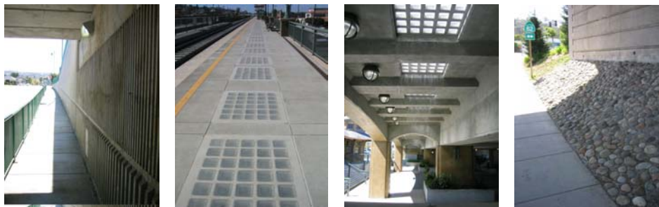
Photos from left to right: Examples of clear line of sight for increased security; glass pavers in platform; ‘skylight’ effect created by glass pavers; rock paving to discourage transient behavior.
