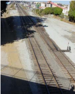
Existing mainline tracks, looking north toward Quint Street. Quint Street freight lead branching off to the right.
