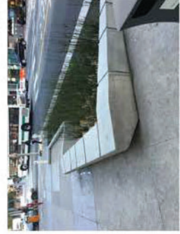
Bulbouts with raingardens help capture and treat stormwater, and can provide seating and other landscaping / habitat opportunities
