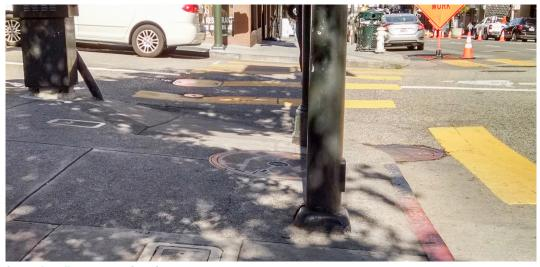
Figure 17. Washington Street West Crosswalk Cross-Slope Exceeds 2 Percent
