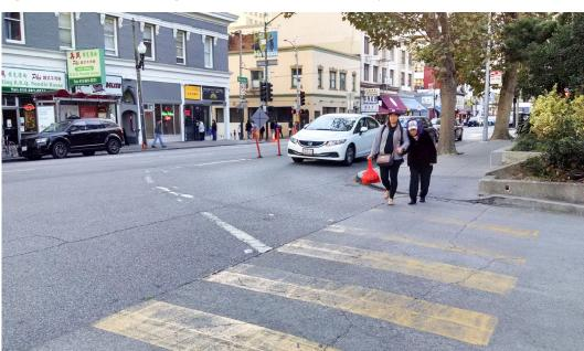
Figure 22. Crosswalk Markings do not Extend to the Curb Ramp Flares
