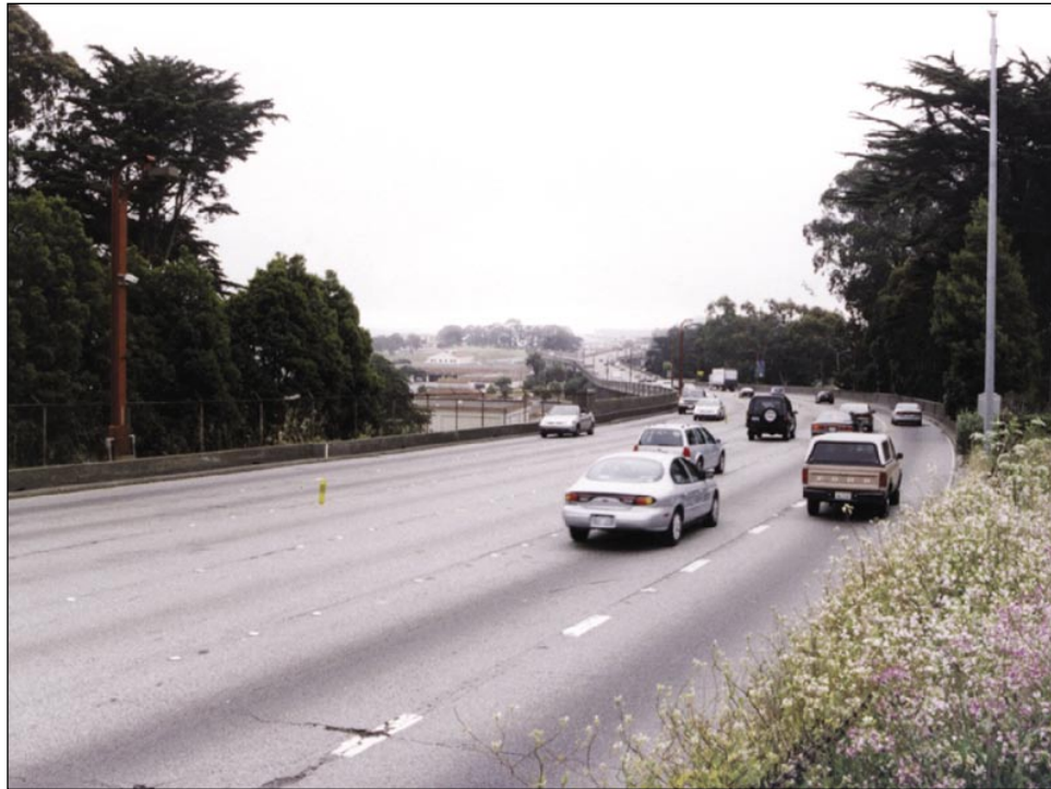
View 13: Doyle Drive at West End of Marina Viaduct, facing east.
