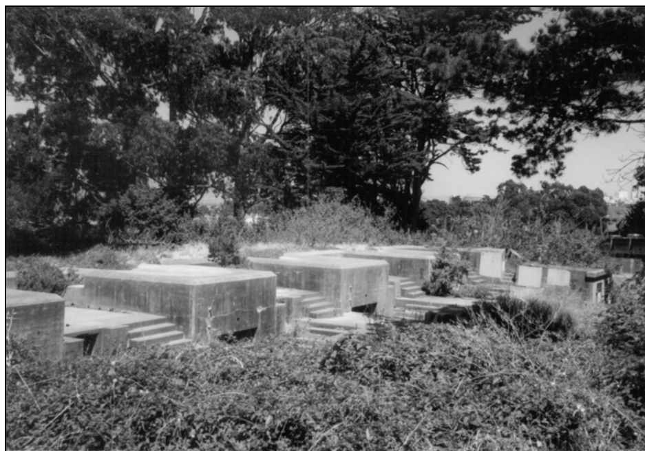
Battery Blaney, camera facing east.
