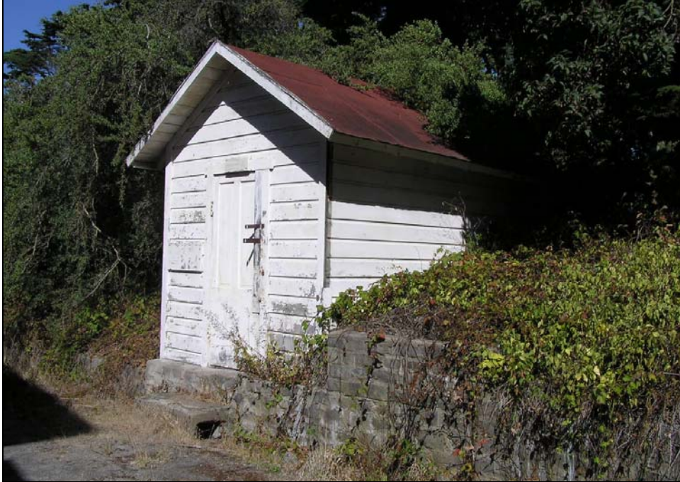
Building 671, camera facing northeast.
