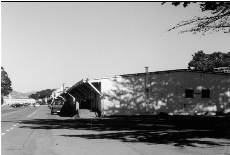
Building 1185, camera facing east.
