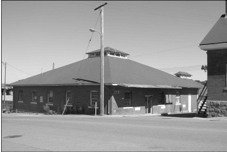
Building 228, camera facing northeast.
