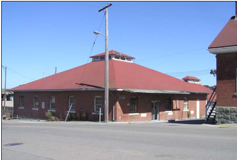
Building 228, camera facing northeast.
