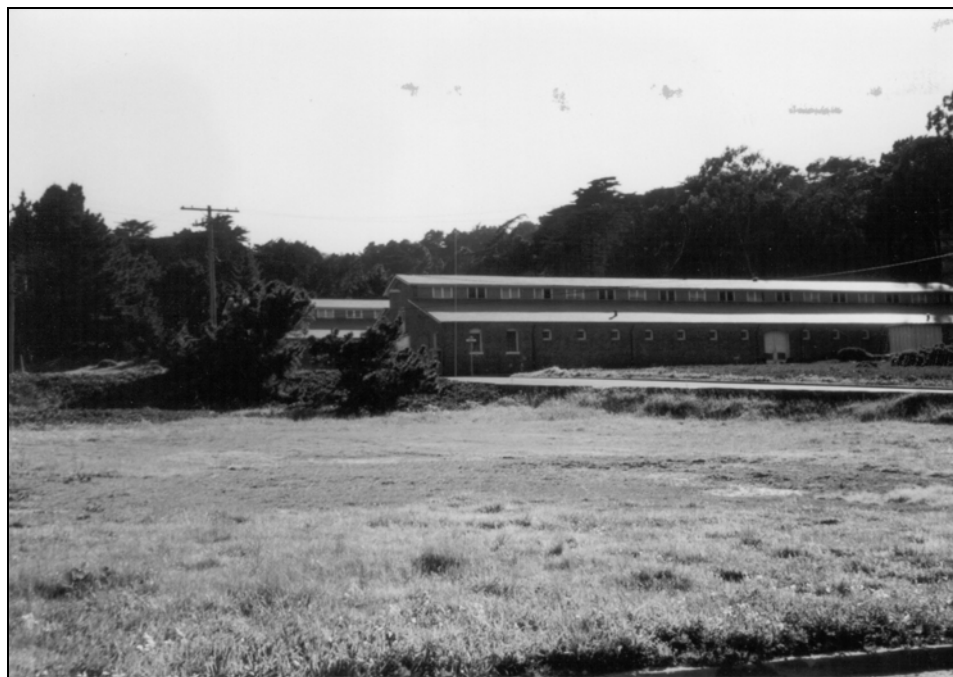
Building 662 and Building 663 (behind), camera facing south.
