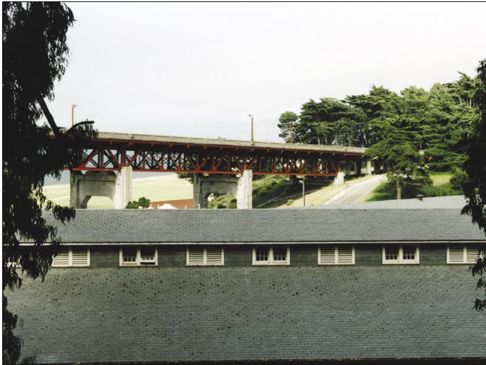
View 10: Stables and Presidio Viaduct, facing northeast.
