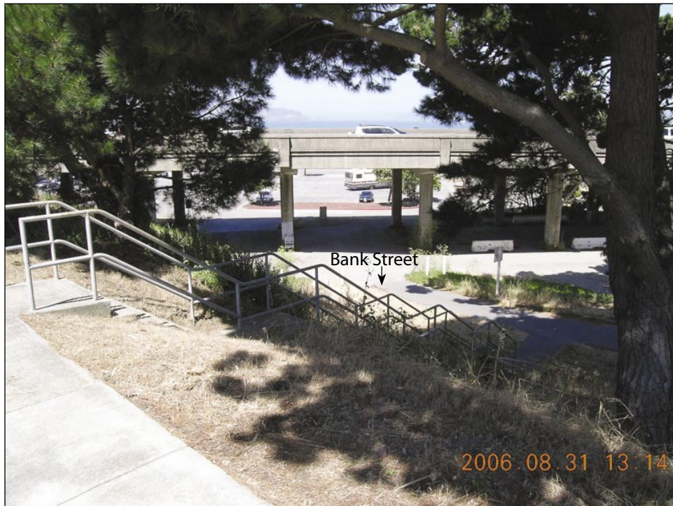
View 23: Marina Viaduct North and West of Building 211, facing north.
