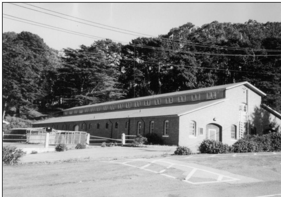
Building 668, camera facing southeast.
