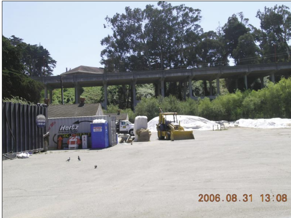
View 21: Marina Viaduct and Buildings 632 and 631, facing south.
