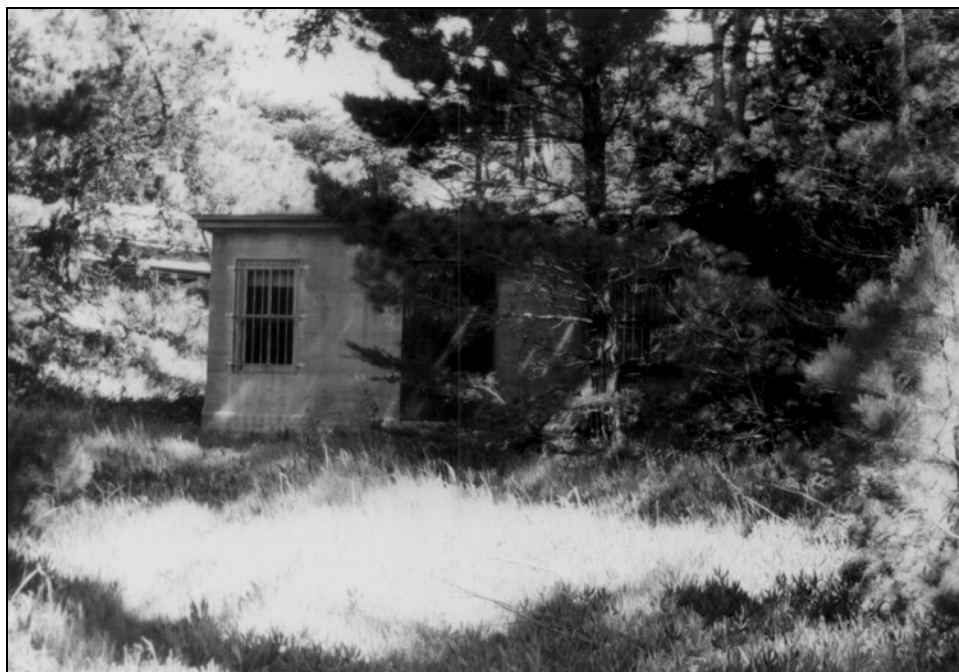
Building 670, camera facing northeast.
