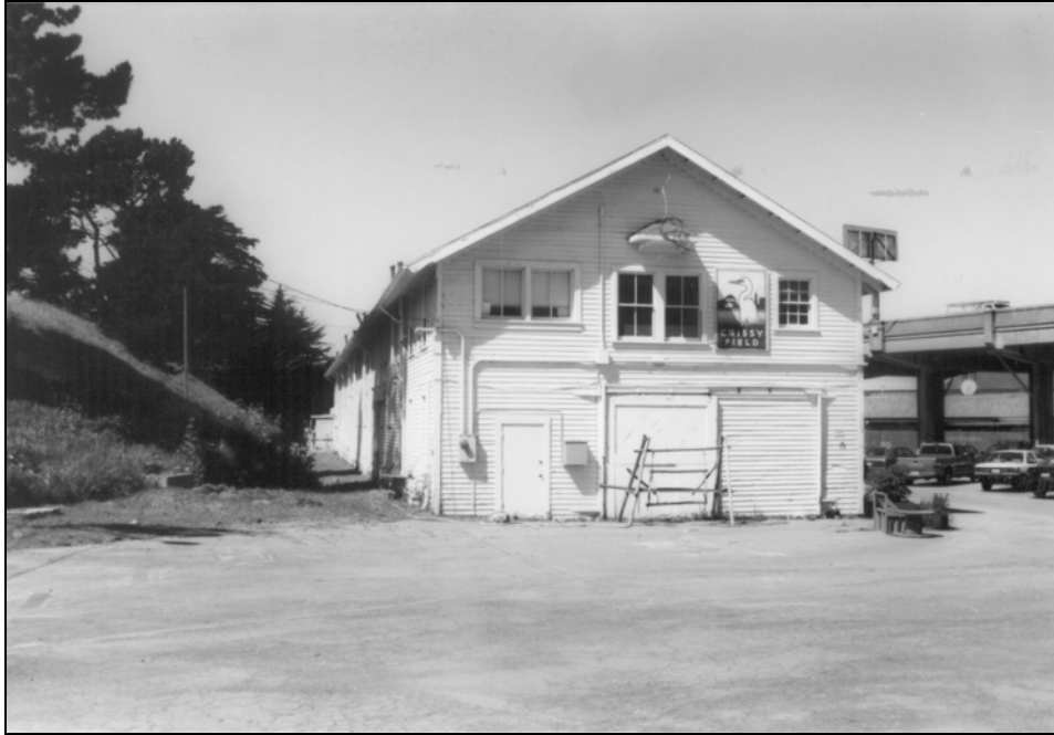
Building 204, camera facing west.
