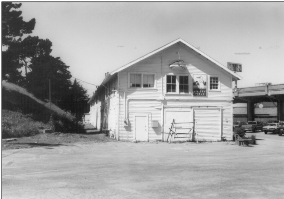
Building 204, camera facing west.
