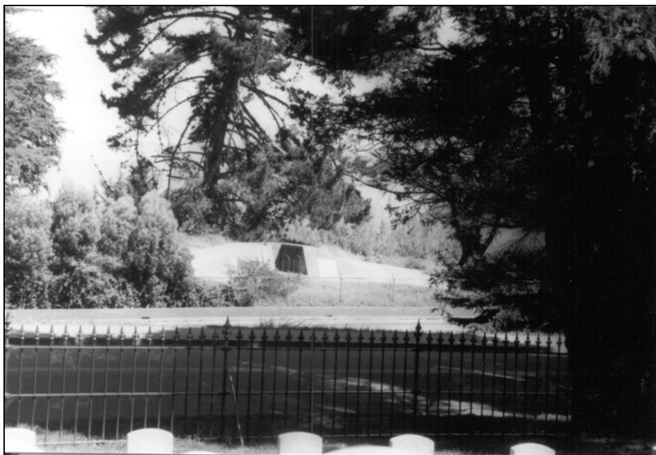
Battery Slaughter as seen across Doyle Drive from National Cemetery, camera facing north.
