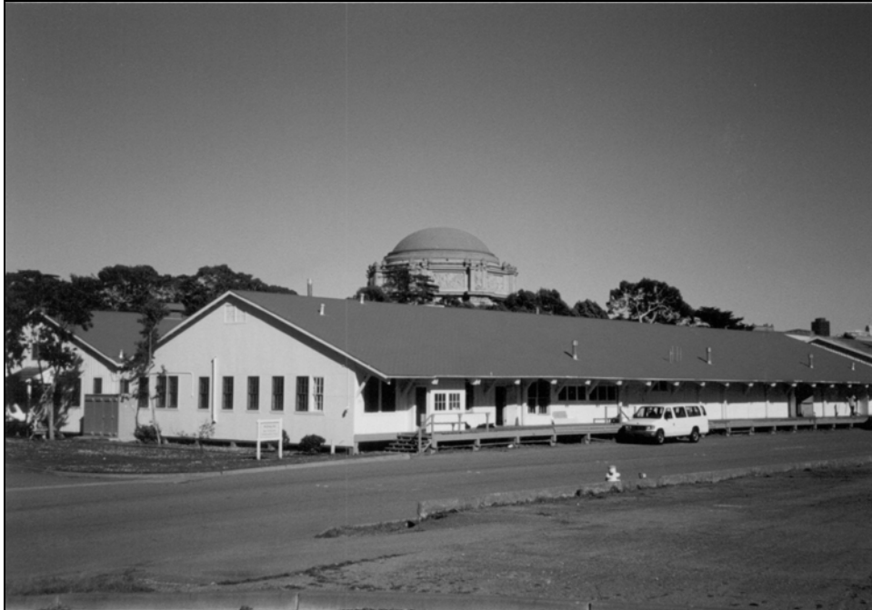
Building 1163 and Building 1167 (behind at left), camera facing east.
