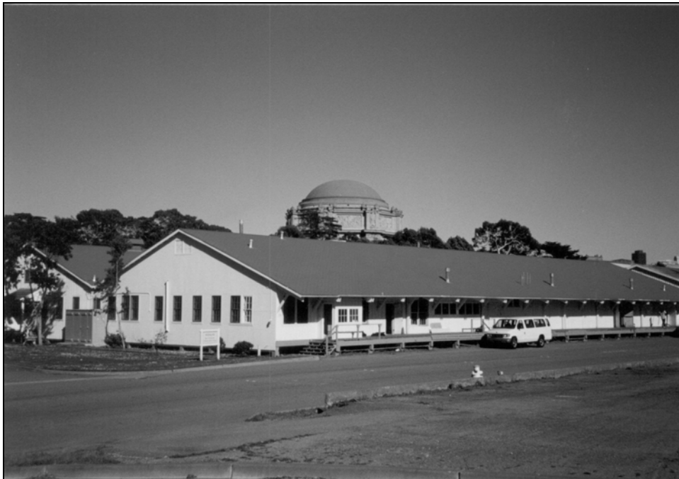
Building 1163 and Building 1167 (behind), camera facing east.
