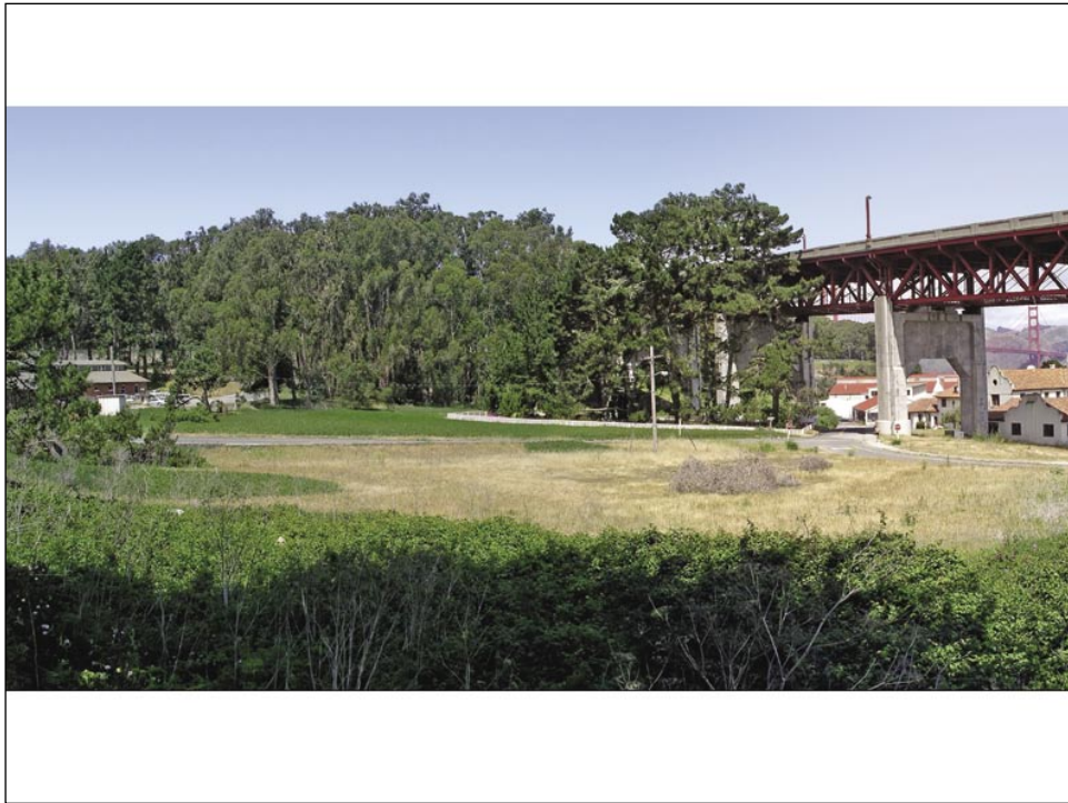
View 17: Presidio Viaduct and Stables Area, facing northwest.
