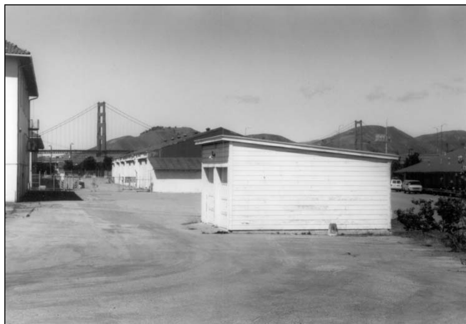
Building 1076, camera facing northwest.
