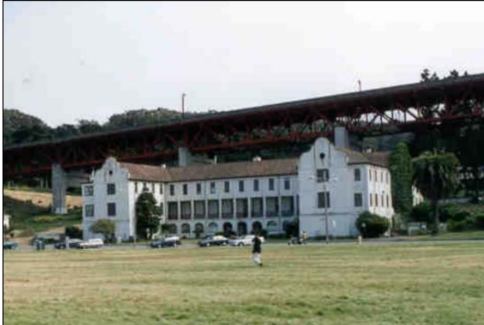
Building 650, camera facing southeast
