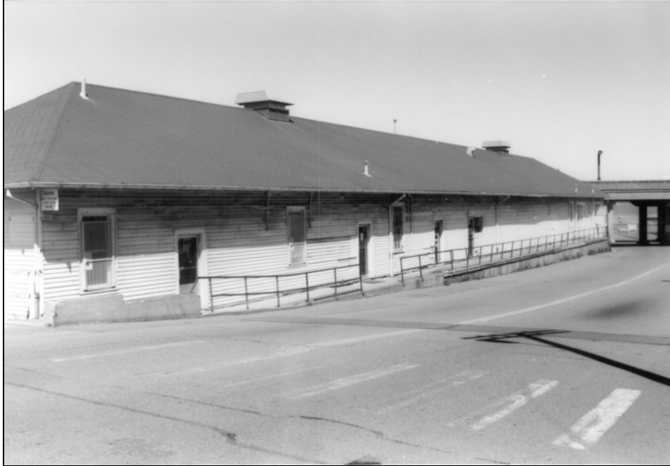
Building 201, camera facing northwest.
