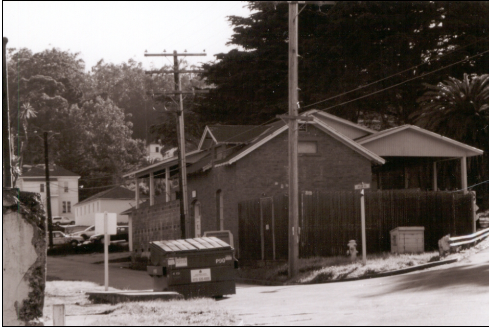
Building 107 with Building 108 behind, camera facing southwest.
