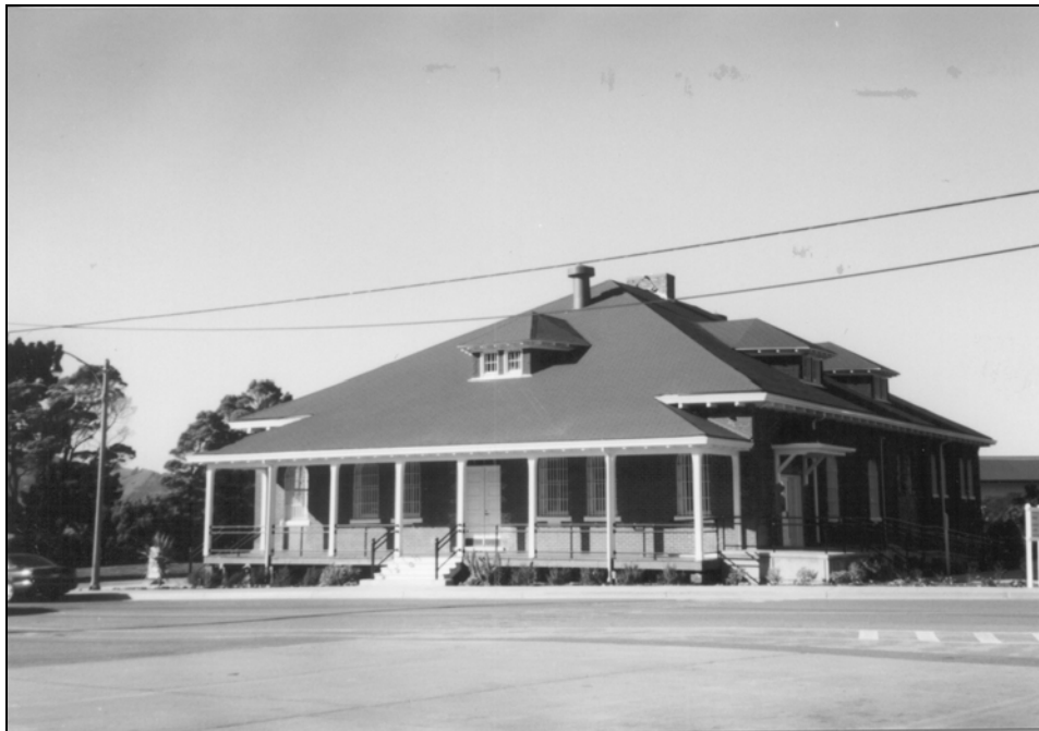
Building 210, camera facing north.
