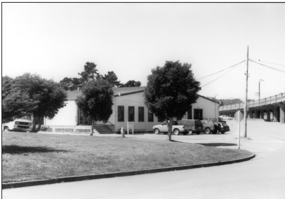
Building 230, camera facing west.
