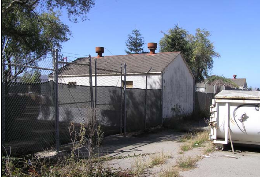
Building 631, camera facing northwest.
