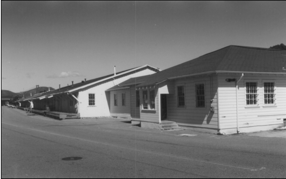
(From L to R) Building 1161 and Building 1160, camera facing northeast.
