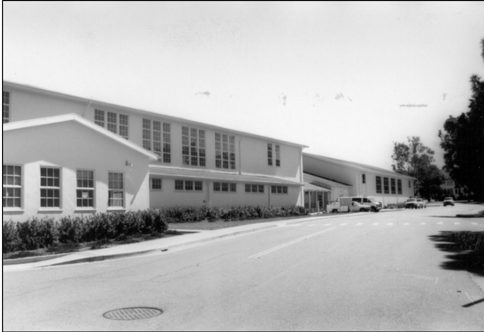
(From L to R) Building 1152 and Building 1151, camera facing east.
