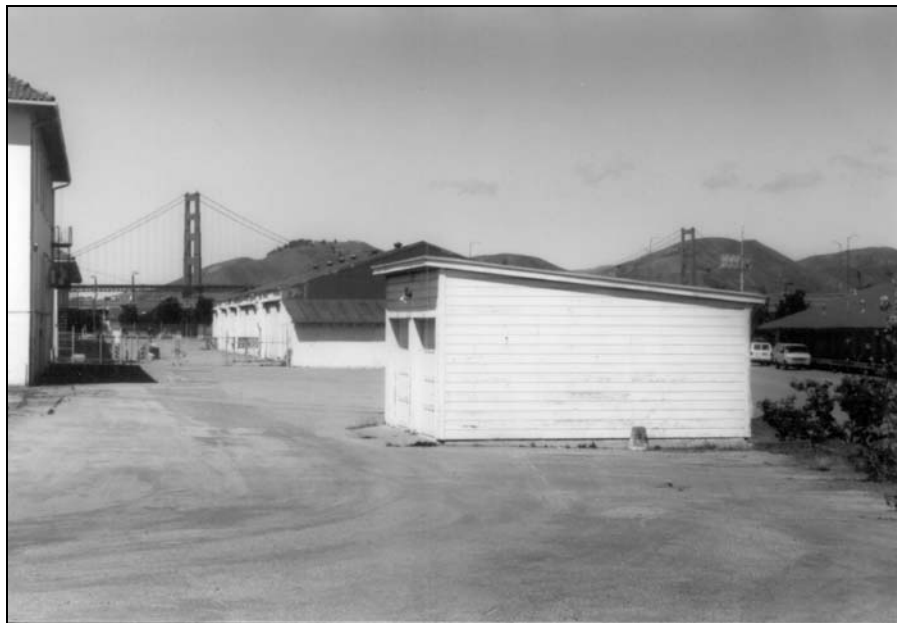
Building 1076, camera facing northwest.
