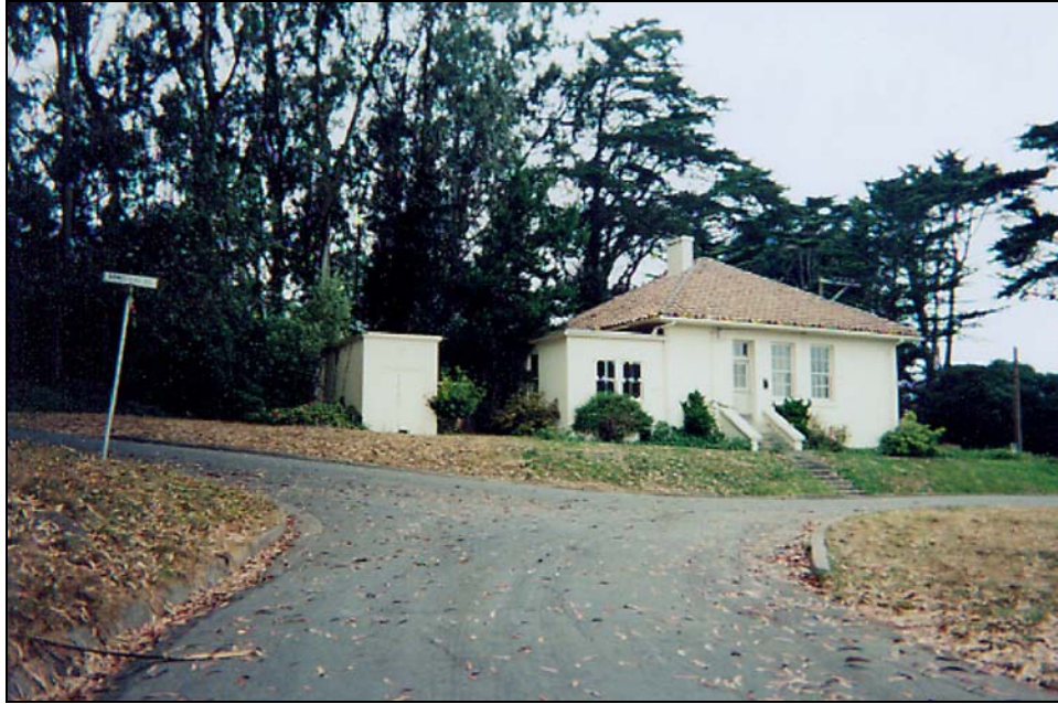
(From L to R) Building 967 and Building 966, camera facing southwest.
