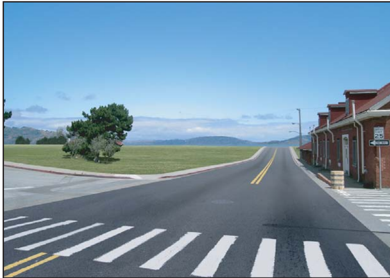
Alt 5: Note loss of Buildings 201 and 204, change in topography, and loss of road network.
