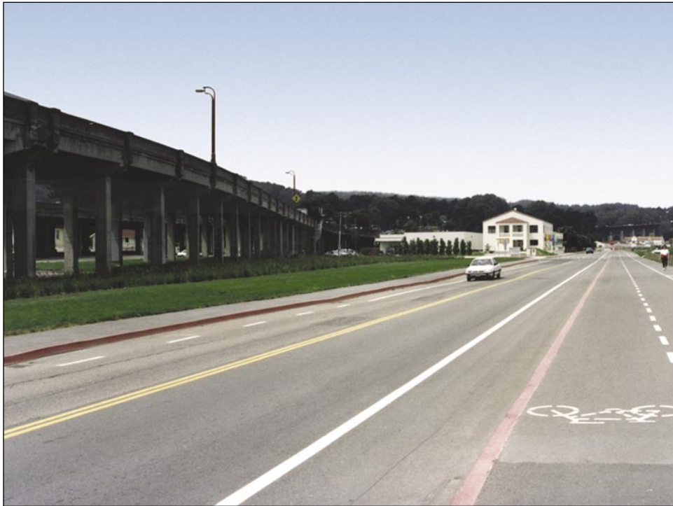
View 7: West End of Mason Street, facing east.
