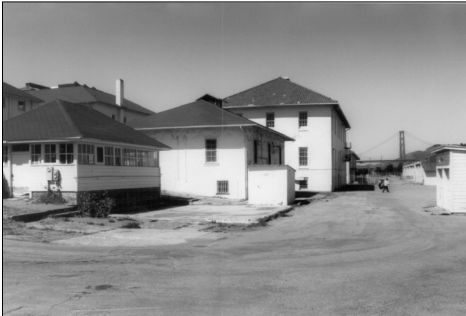
(From L to R) Buildings 1056, 1059, and 1060, camera facing west.
