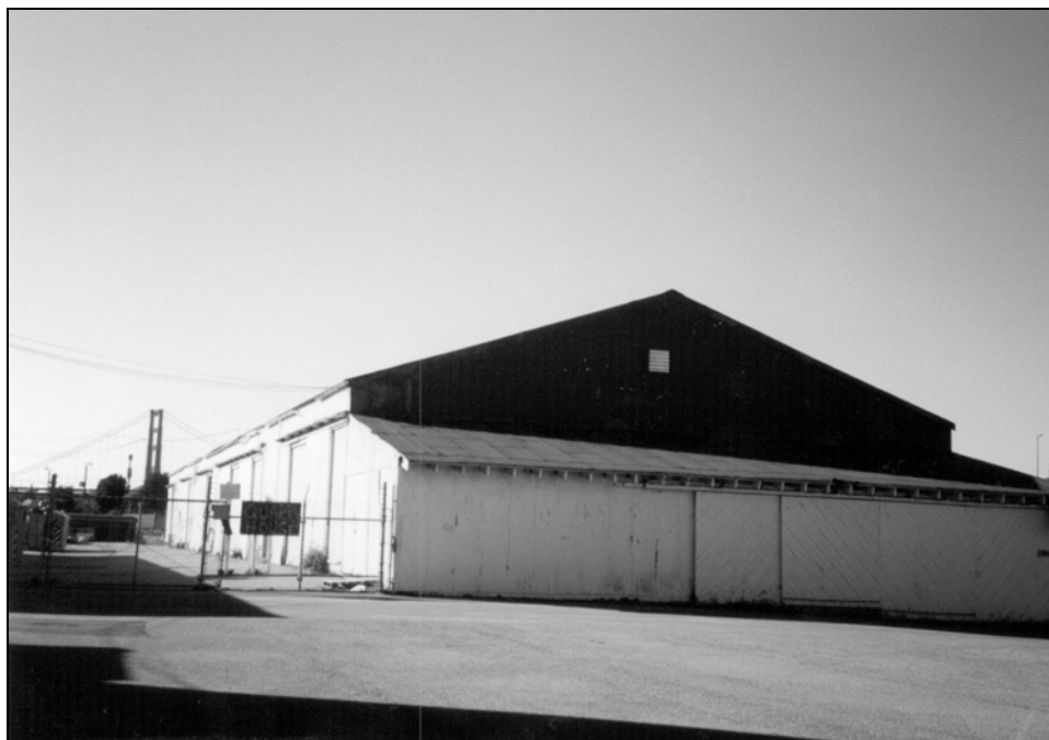
Building 1063, camera facing northwest.
