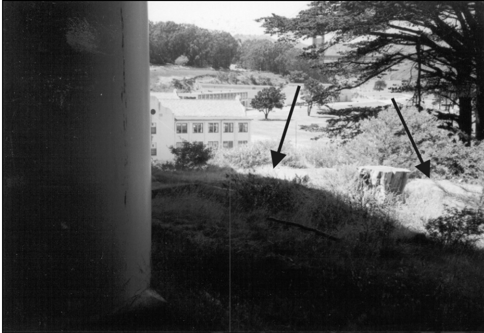
Battery Baldwin remains (indicated by arrows), adjacent to Presidio Viaduct east abutment, camera facing northwest.
