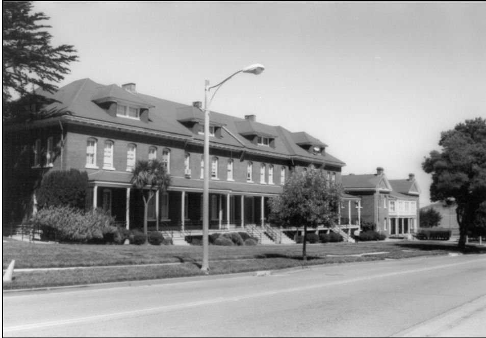
(From L to R) Building 105 and Building 106, camera facing north.
