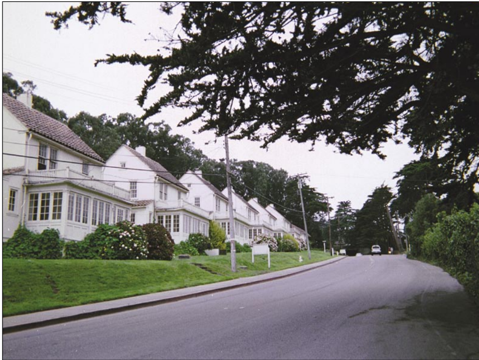
View 20: Pilot's Row, facing southwest.
