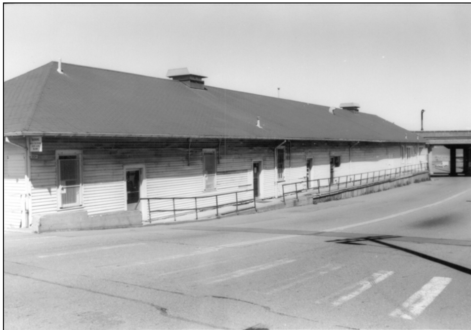
Building 201, camera facing northwest.
