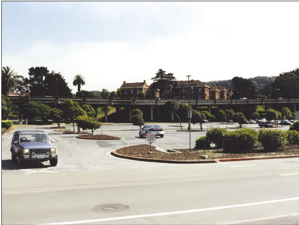
View 8: Marina Viaduct and Main Post Buildings, facing southwest.
