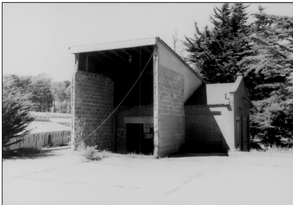
Building 669, camera facing northwest.
