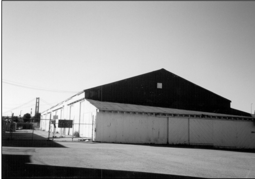
Building 1063, camera facing northwest.
