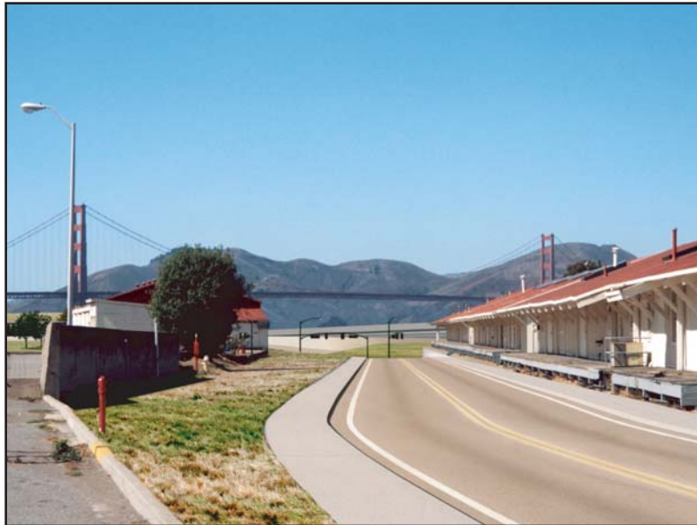
Alt 5 - Note Absence of Building 230 at Left
