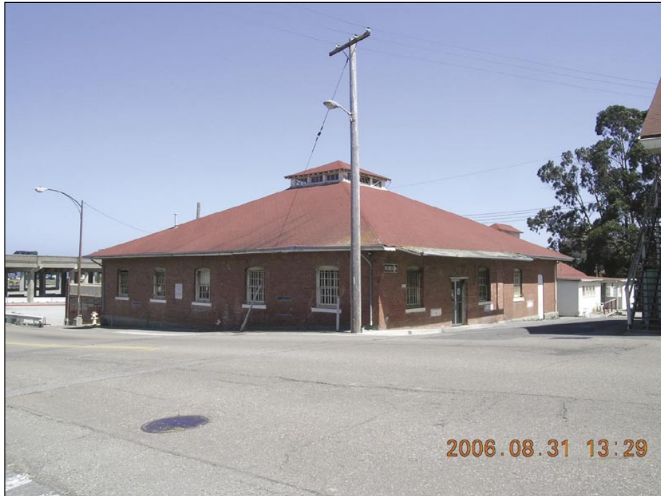
View 22: Building 228, facing northeast.
