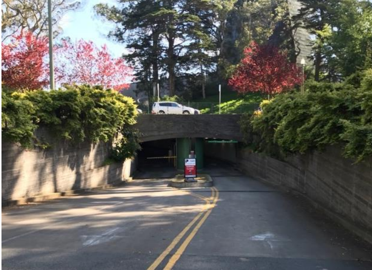
Figure 9 – Connecting tunnel between the two halves of the Concourse Parking Garage
