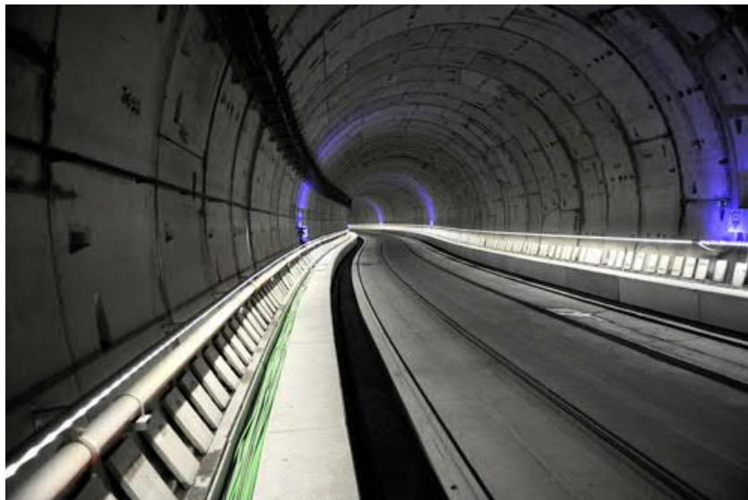
Figure 5: Inside the Atocha Chamartin Tunnel
