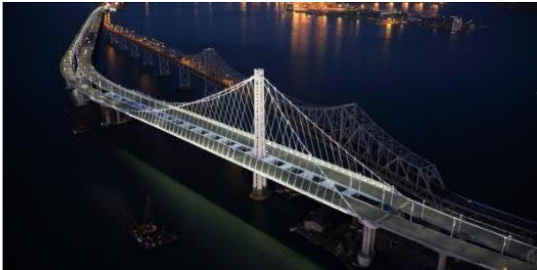
Figure 20: New East Span of the San Francisco-Oakland Bay Bridge
