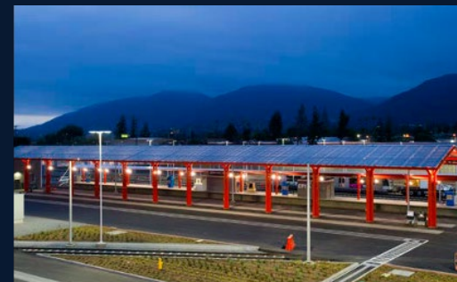
FOOTHILL GOLD LINE LIGHT RAIL EXTENSION PHASE 2A DESIGN LOS ANGELES, CA
