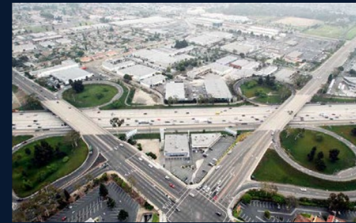
I-405 IMPROVEMENT PROJECT (SR-73 TO I-605) PA/ED AND DB PROGRAM MANAGEMENT ORANGE COUNTY, CA
