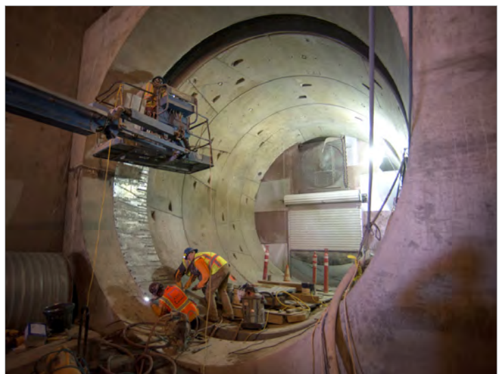
Tunneling work was completed on time and under budget.
