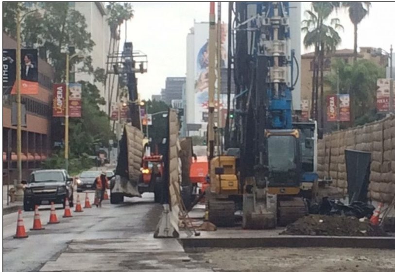
Figure 7-16. Example of Footprint Required for Jet Grout Operations from Surface and Associated Traffic Control (LA Metro Purple Line)
