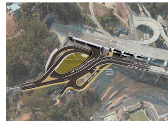
The Southgate Road Realignment project is 75% complete as of the end of 2021
