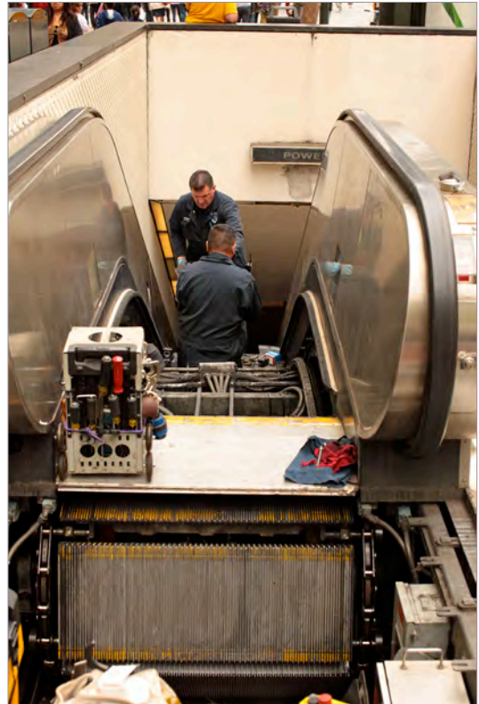
▲ Prop K half-cent local transportation sales tax funds help pay for station repairs.
