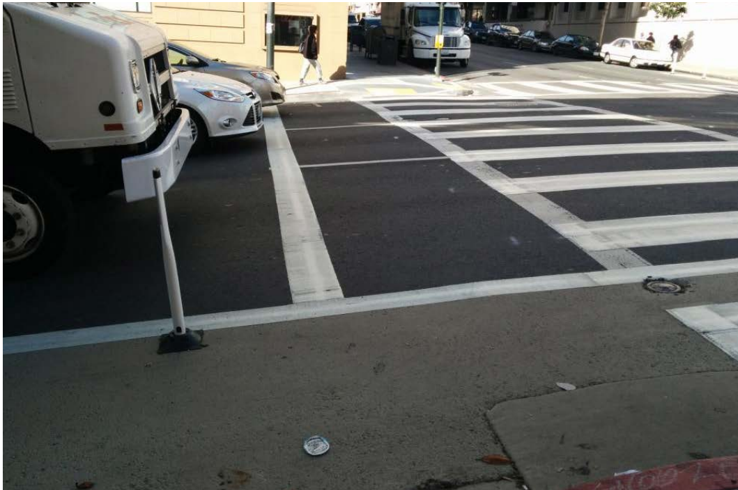
Figure 3-11. Advanced limit lines are painted lines before crosswalks to signal to mark where drivers should stop and prevent them from encroaching onto the crosswalk.
