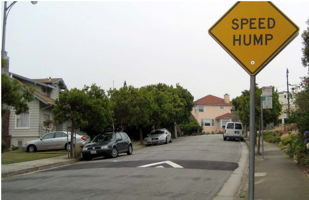
Figure 3-1. Speed humps reduce vehicle speeds
