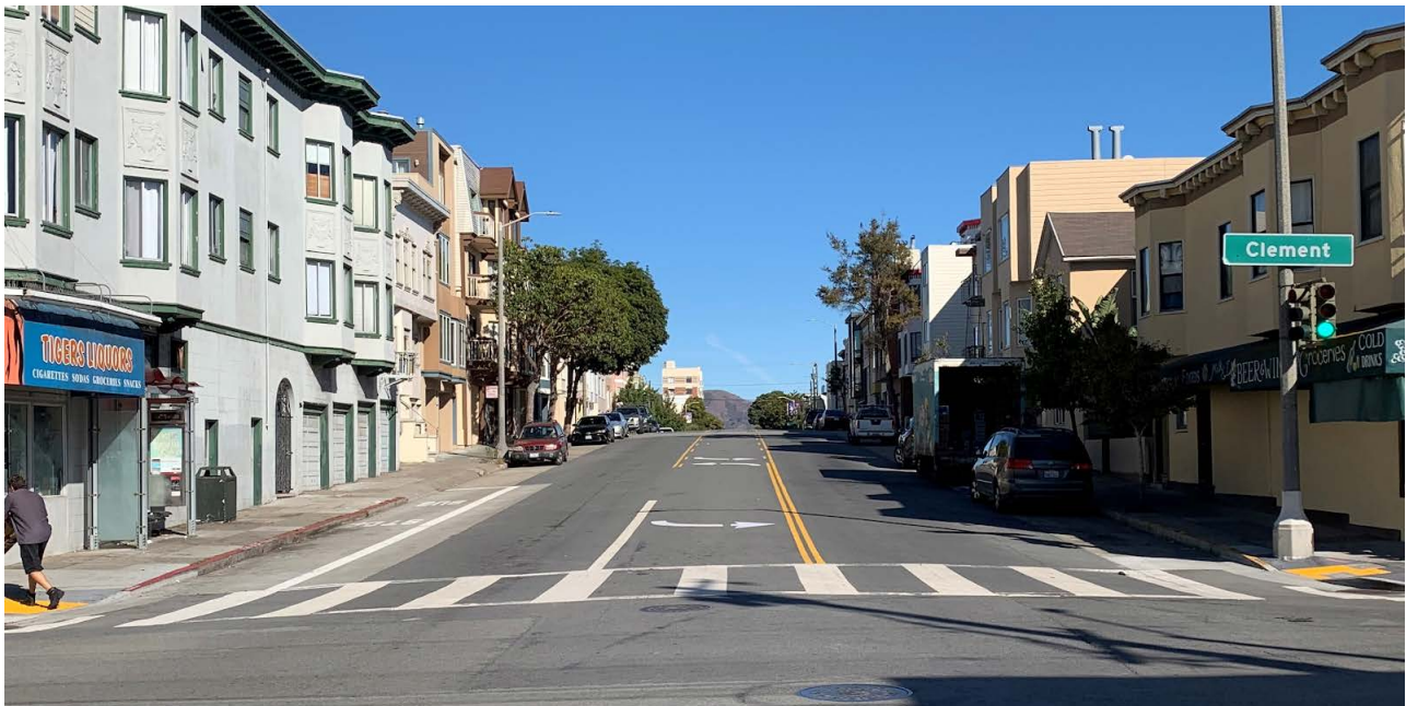
Figure 3-12. A road diet converts a four-lane street to a three-lane street with a center turn lane.
