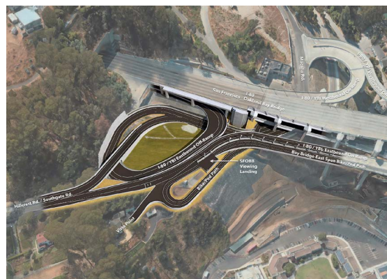
The Southgate Road Realignment project is nearly complete as of the end of 2022.
