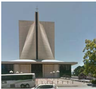
St. Mary's Cathedral is located on Geary Boulevard at Gough Street
