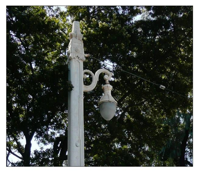
Photograph 10: Detail showing exterior wiring inserted in Pole 264, with original finial and 1936 bracket and modern luminaire, Van Ness Avenue between Greenwich and Filbert streets, 4/1/2009.
