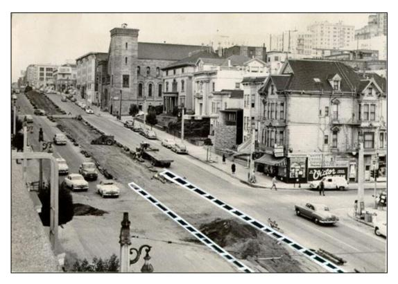
Photograph 27: Track removal on Van Ness Avenue at Vallejo Street in 1952. Note contrasting color of finials and brackets. Also, the result of the WPA street widening (sidewalk narrowing) project is still visible in different color of pavement along sidewalks. Photograph courtesy of San Francisco Public Library Historical Photograph Collection.
