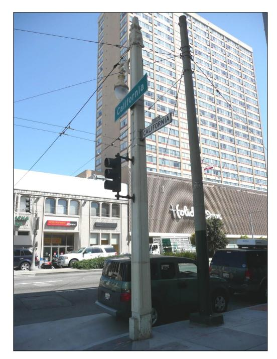
Photograph 12: Alterations to Pole 157, including insertion of traffic signal equipment, signage added, base removed, and modern metal pole installed adjacent. Located southwest corner of Van Ness Avenue and California Street, 4/1/2009.
