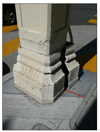
Photograph 15a and 15b: Example of fiberglass replacement base (this one with foliated detailing), no access doors, Pole 308, at the southeast corner of Van Ness and Bay, 4/1/2009.
