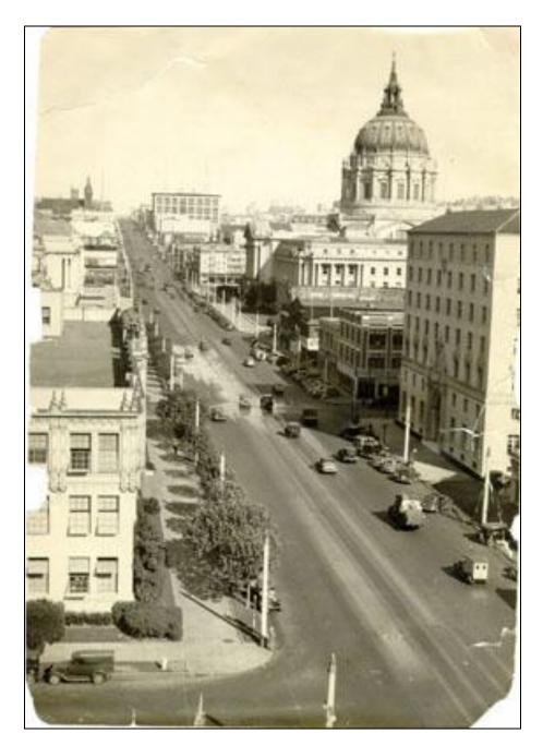
Photograph 24: Van Ness Avenue looking north from Fell Street in 1935. This photo was taken just before the 1936 WPA project and the original pairs of lights are still in place. The poles line the corridor with their original and uniformly uncluttered aesthetic. Photograph courtesy of San Francisco Public Library Historical Photograph Collection.
