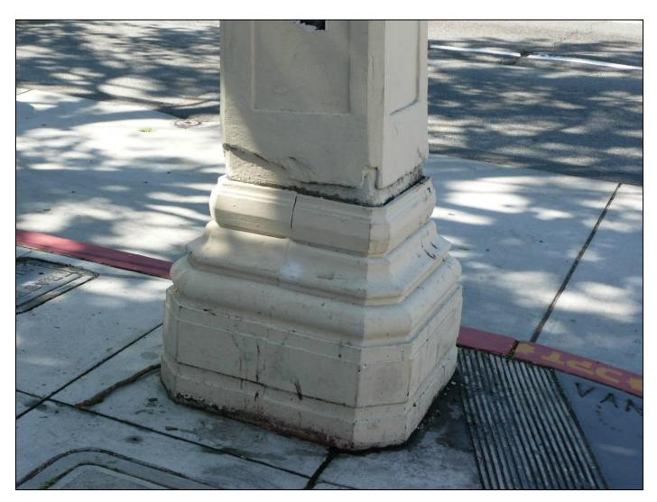
Photograph 9: Replacement fiberglass base without foliated details or access doors, Pole 228, southeast corner of Van Ness Avenue and Vallejo Street, 4/1/2009.
