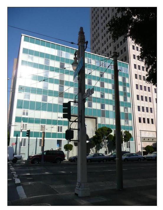
Photograph 19: Pole 17, with insertion of traffic signal equipment, signage added, and installation of adjacent modern metal pole, Van Ness Avenue and Hayes Street, 4/1/2009 (shown in Photograph 18 above).
