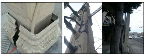
Photos 31-33. Damaged and leaning OCS support pole/streetlights.
